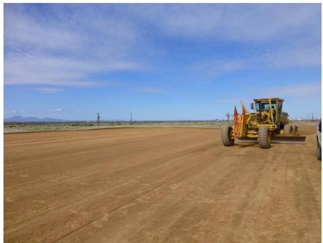
February 21, 2013: CGRC Flyers' RC field being built. (Photo courtesy Alan Friedman.)
